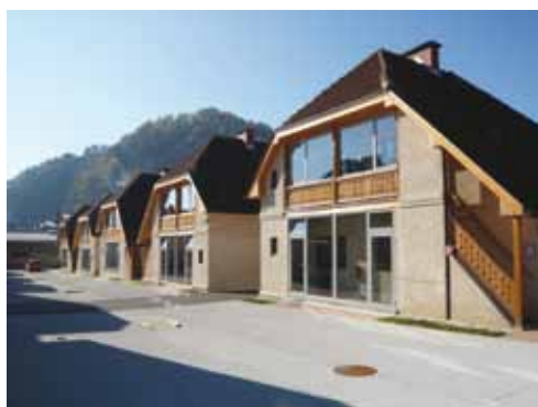
Figure 4. Slovenians being proud that 63 % of their country is covered with forests find it difficult to accept the newly “renewed” municipal colony in Trbovlje. Never before has this place seen houses that were glazed with metal builder’s joinery. The reason for the undertaking of such renovation procedures was the belief that the new renovation “additions” should be easily identifiable. Unfortunately this became the opposite of the intended, because, now, after the renovation, the “colony” seems as a series of modern summer houses from somewhere in the upper Sava Valley (photo: V. Hazler, 2010).
